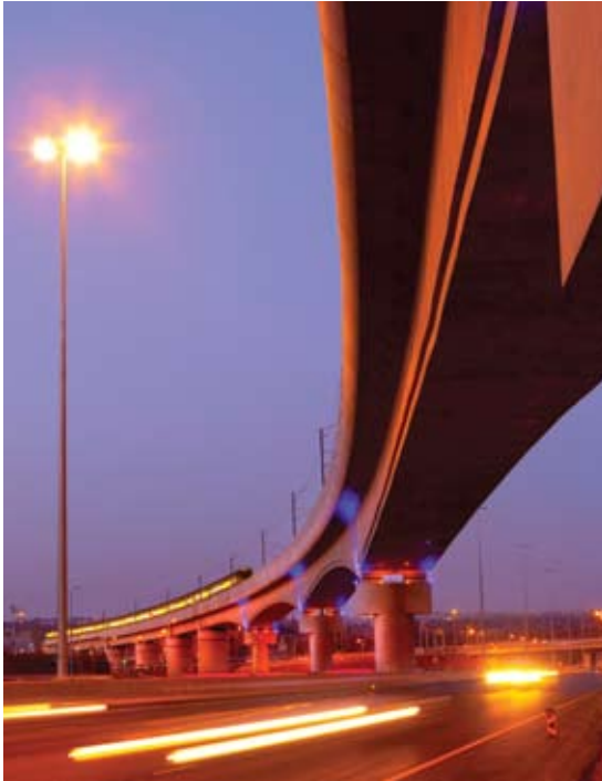
COVER Gautrain crosses the N1 Highway between Tshwane and Johannesburg
